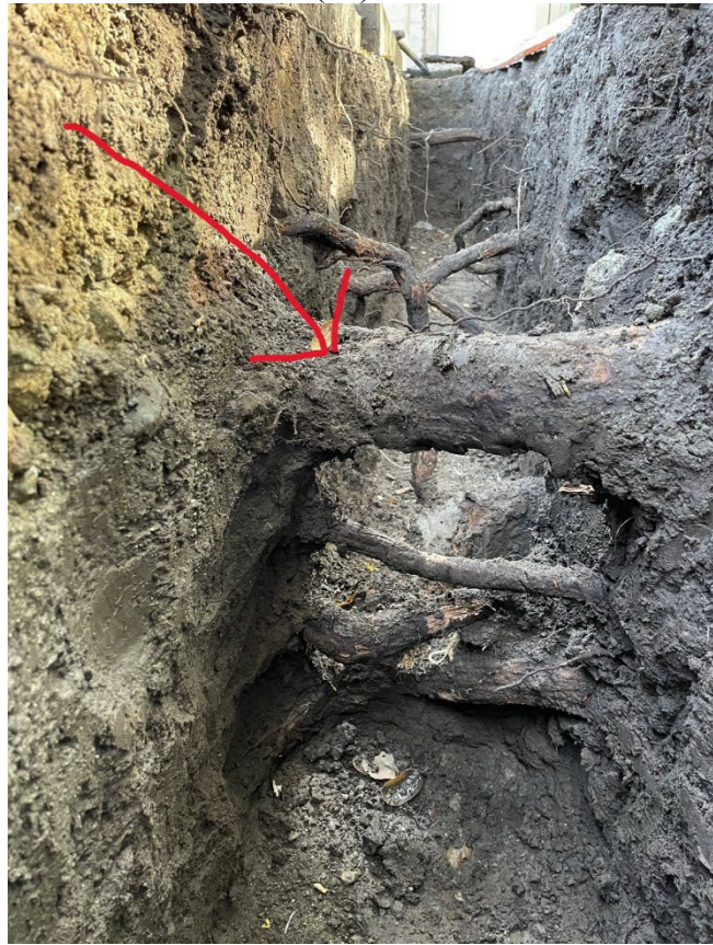
Showing largest root (3.2") to be cut
