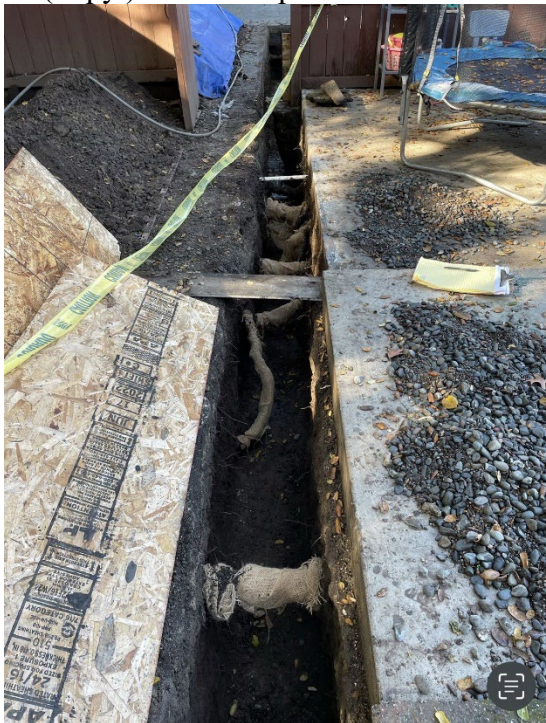
Showing encountered roots within the Landscape area wrapped in burlap
